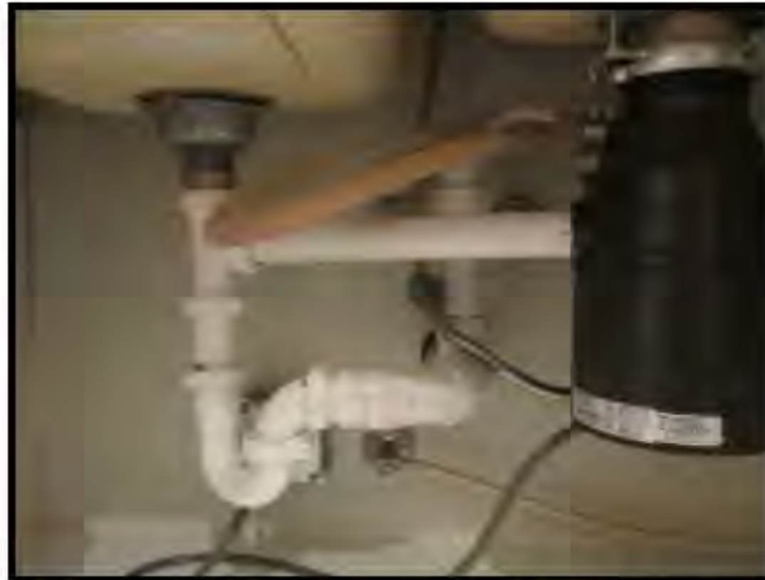
Kitchen plumbing, no signs of leaks at time of inspection
