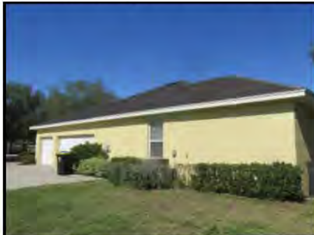
The exterior drainage is generally away from foundation.
