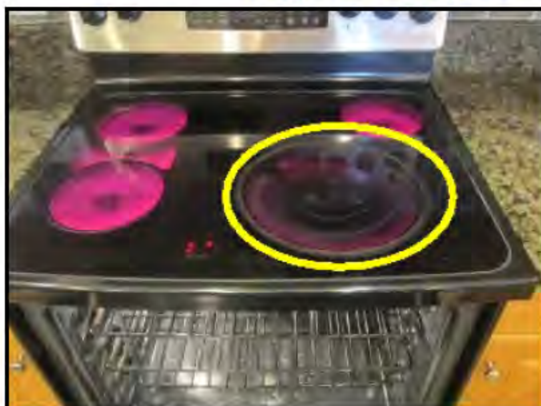
Front right element did not appear to be working fully at time of inspection, May need replaced
