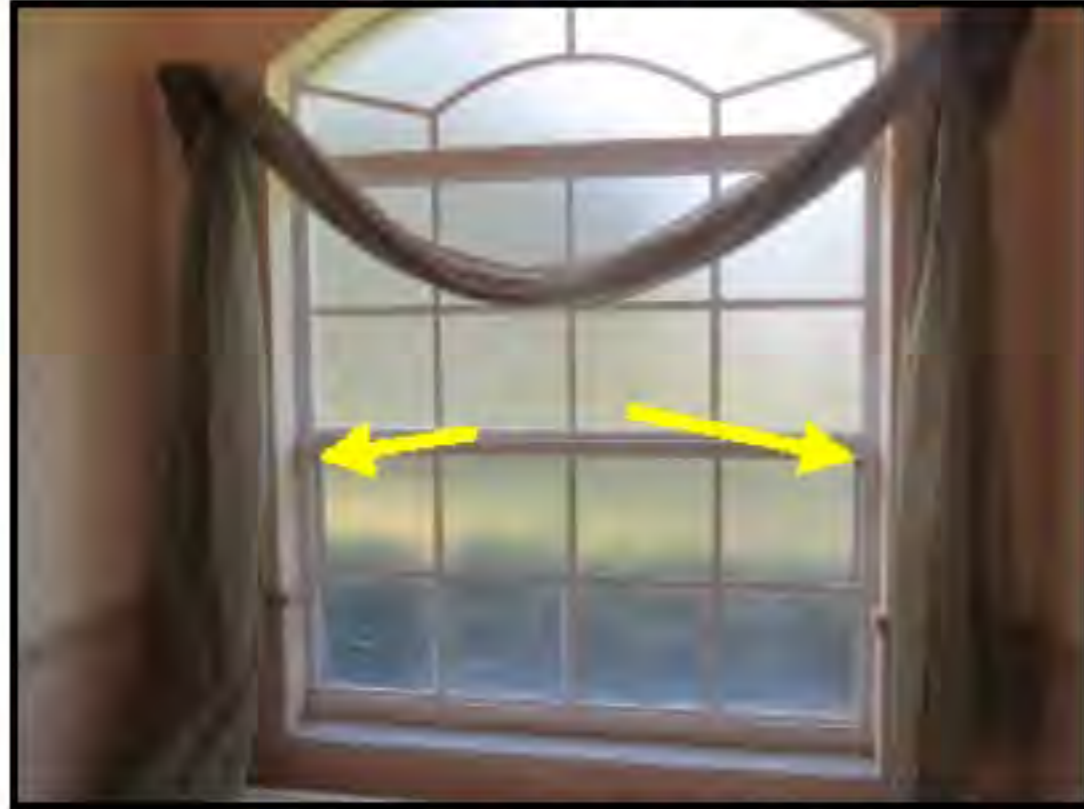
Broken window balance noted in Master Bathroom, wont stay in the open position
