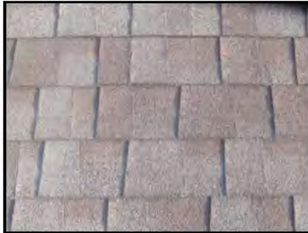
Roof in within its useful life, satisfactory condition
