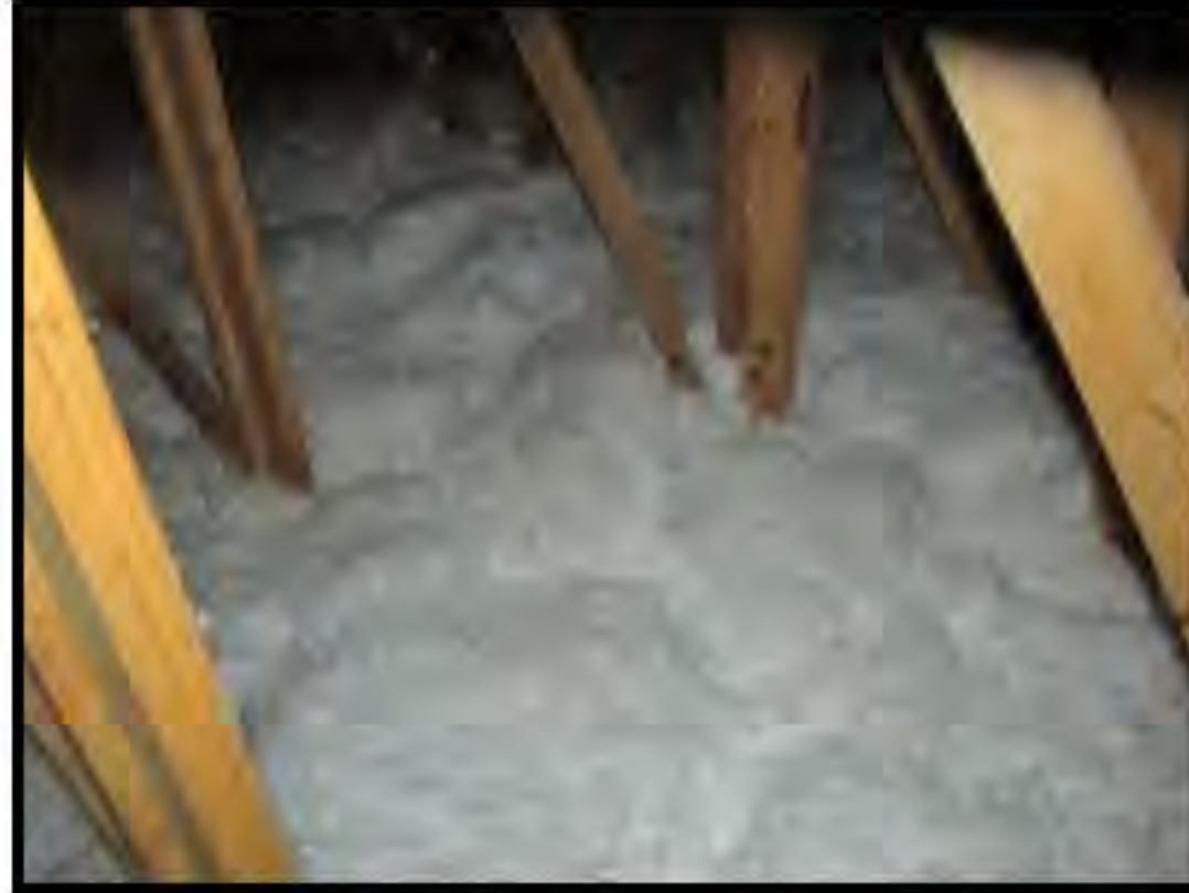
Insulation appears adequate.
